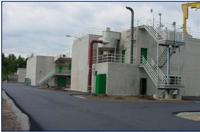
Headworks Building (grit removal, secondary screening, anoxic basins)
