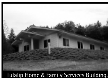
Tulalip Home & Family Services Building.
